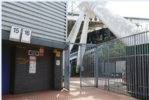
Figure 18 Accessible Entrance next to Turnstile 16
