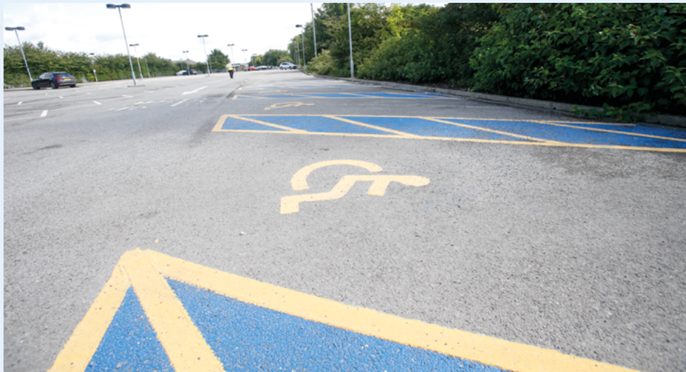
Figure 2 Town Avenue car park disabled parking bays
